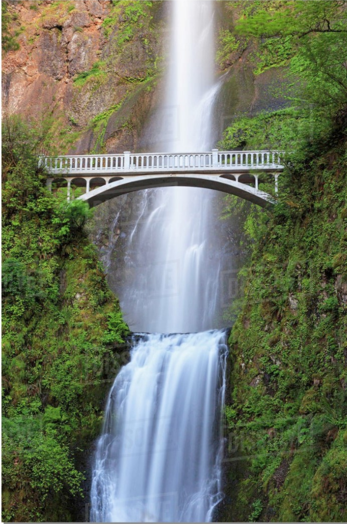
Benson Bridge (pictured here) is located at Multnomah Falls, Oregon. The bridge was completed in 1914 and is a 45-foot high reinforced-concrete arch pedestrian bridge over the lower Multnomah Falls near the Historic Columbia River Highway. The Multnomah Falls is the most visited tourist location in Oregon each year. The entire span of the Multnomah Falls makes it the fourth longest waterfall in the U.S. at over 542 feet over three basalt falls.
